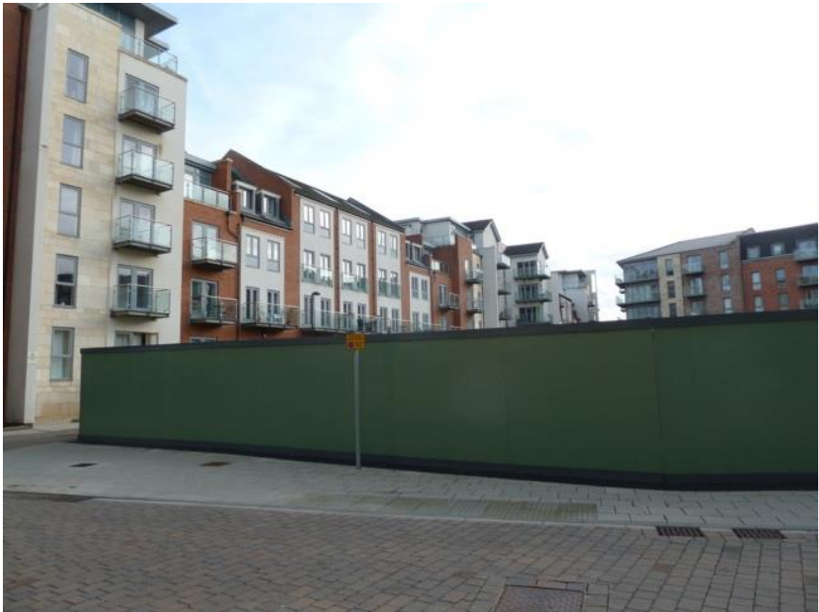
Phase 1 housing seen beyond hoarding round Block D (John Stevens, 2023).
