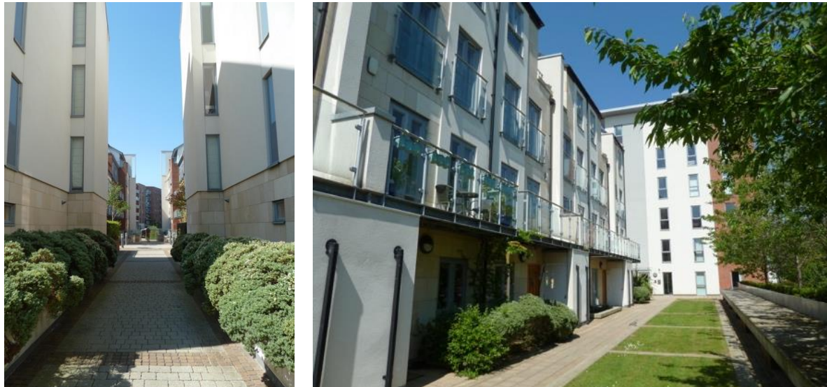
The view west along the pedestrian access to Phase 1 (both John Stevens, 2023).
