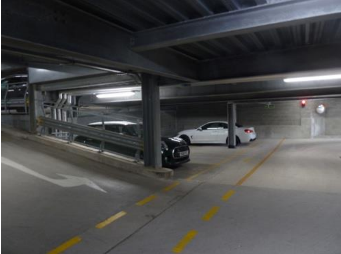
Inside the multi-storey car park at Bellerby Court. (John Stevens, 2023).
