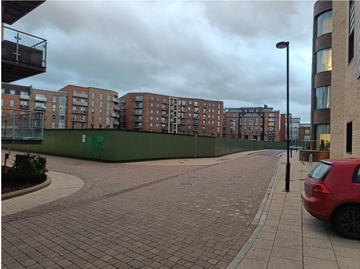
Perimeter massing of Leetham House (left), Bellerby Court (central) and St John Central (right) visually combining as defensive in nature and claustrophobic (Duncan Marks, 2024).
