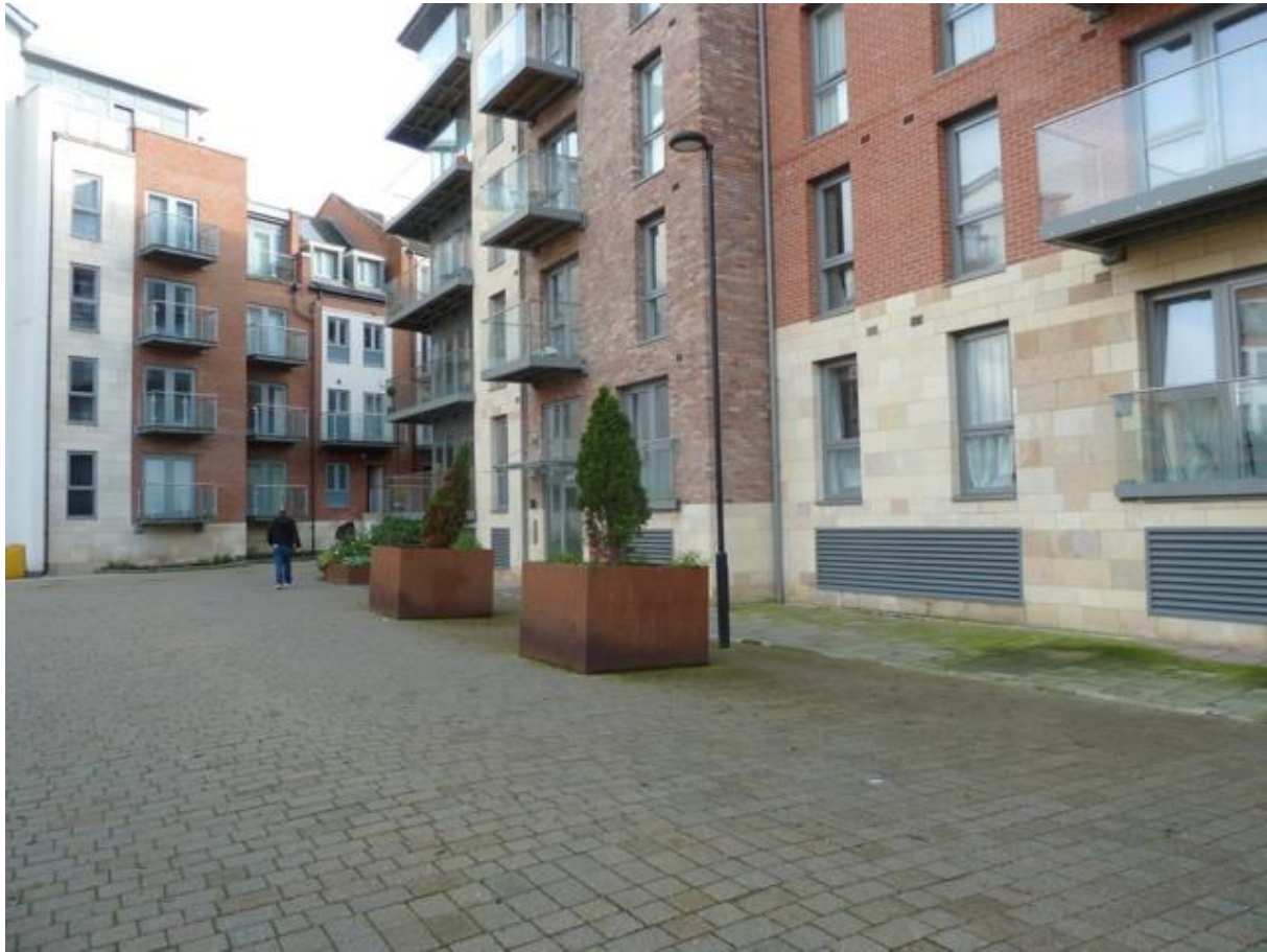
Unimpressive landscaping outside Leetham House (John Stevens, 2023).
