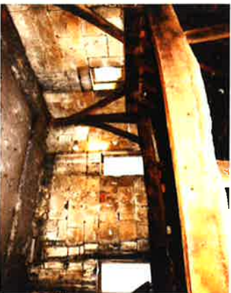
The roof-top room with 'battlements' incorporated into the walls
